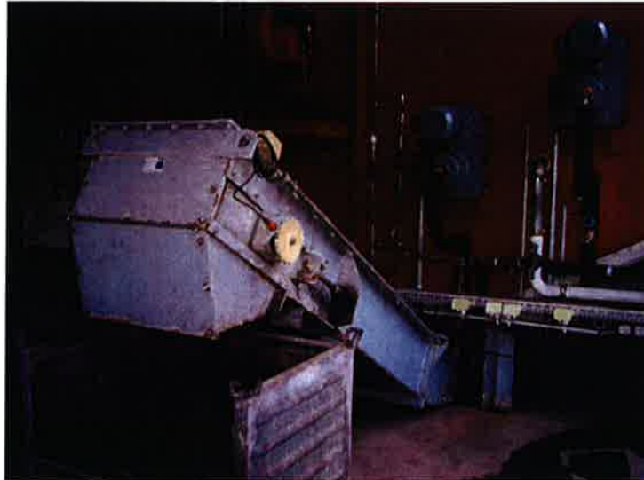
Figure 2: CCC Bottom Ash System
